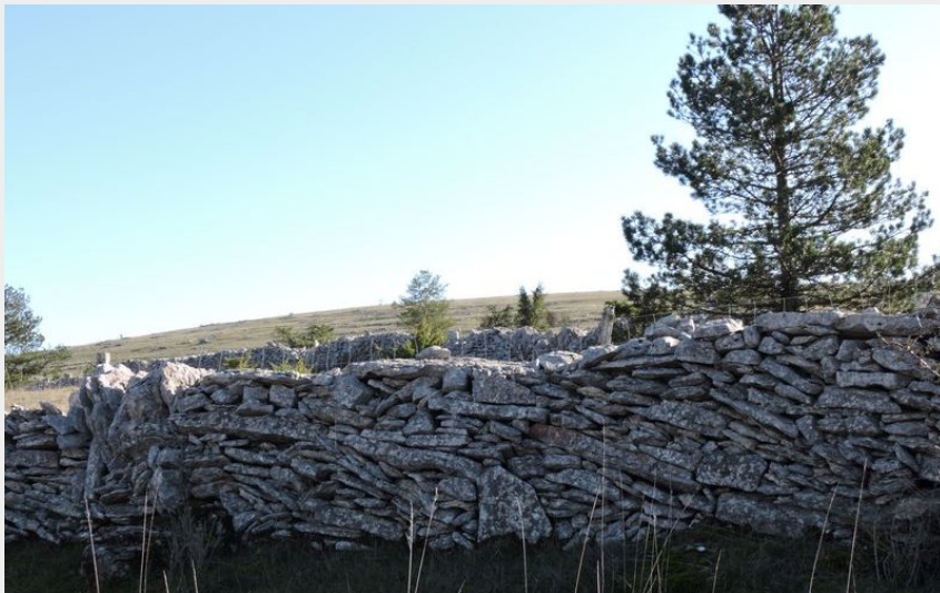
Murets (© OTGCC nc)
