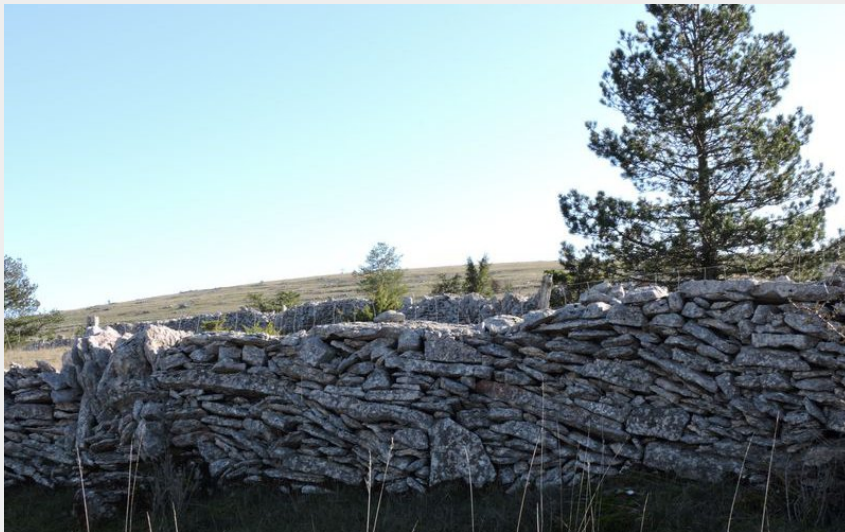
Murets (© OTGCC nc)
